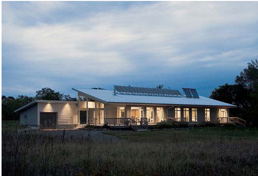
County Trail House
