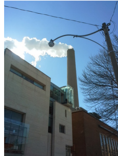
UofT Co-Gen Plant
